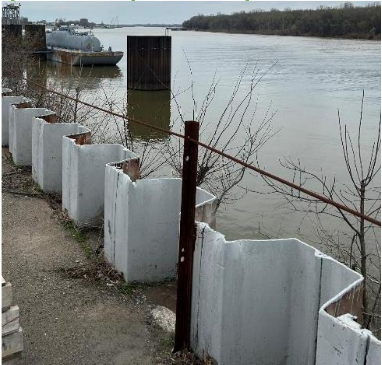
Figure 54: Concrete Loading Zone and Still Retaining Wall at Port of Paducah, KY
