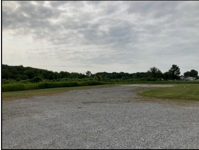
Figure A.4. Unsurfaced road in Union County.
