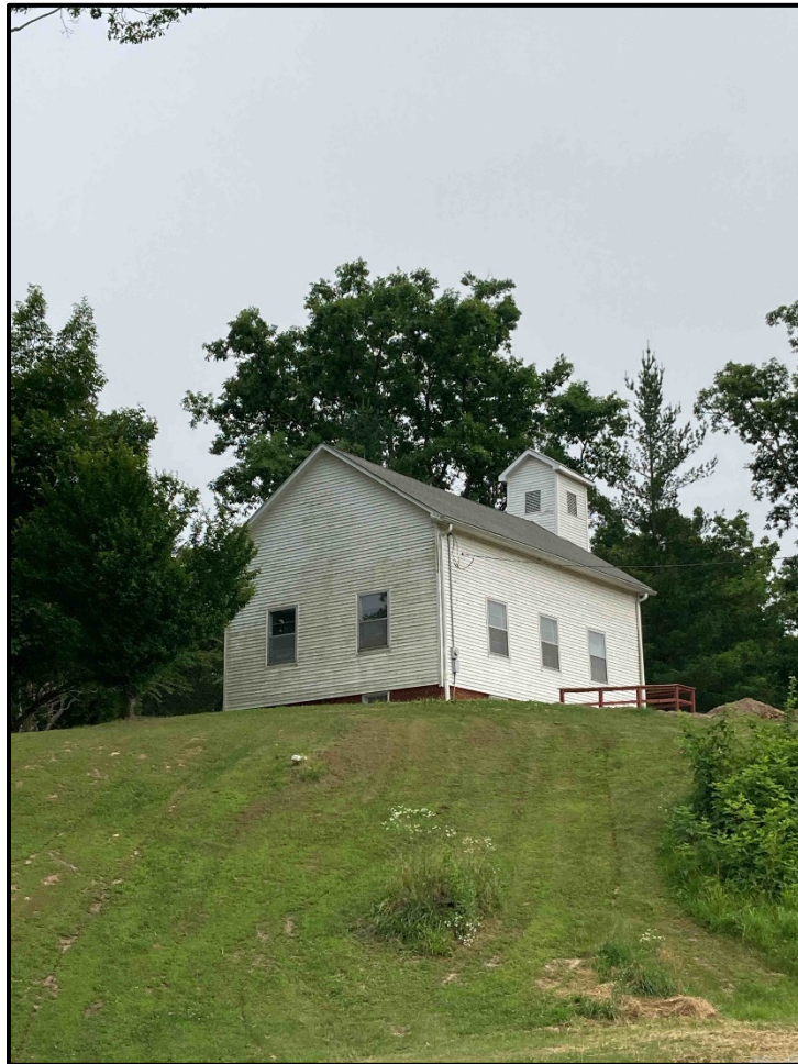
Figure D.26. Values at risk including churches are common scattered in the interface. Most have good defensible space.
