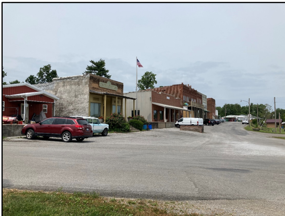
Figure D.17. The community of Alto Pass has a cluster of values at risk, including tourist resources like restaurants and gift shops.
