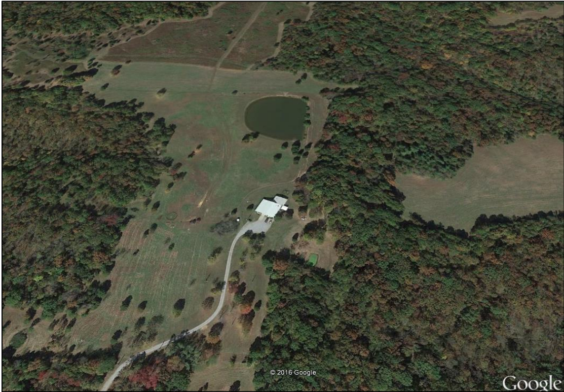
Figure 47. Home with good defensible space, access, turnaround space and pond.
