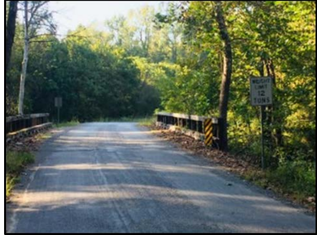
Figure 3.15. Bridge close to the Iron Furnace with weight limit.
