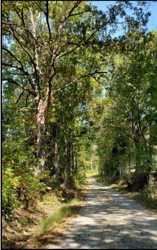
Figure 4.29. Finneyville Road (840 N) is unsurfaced and very narrow.
