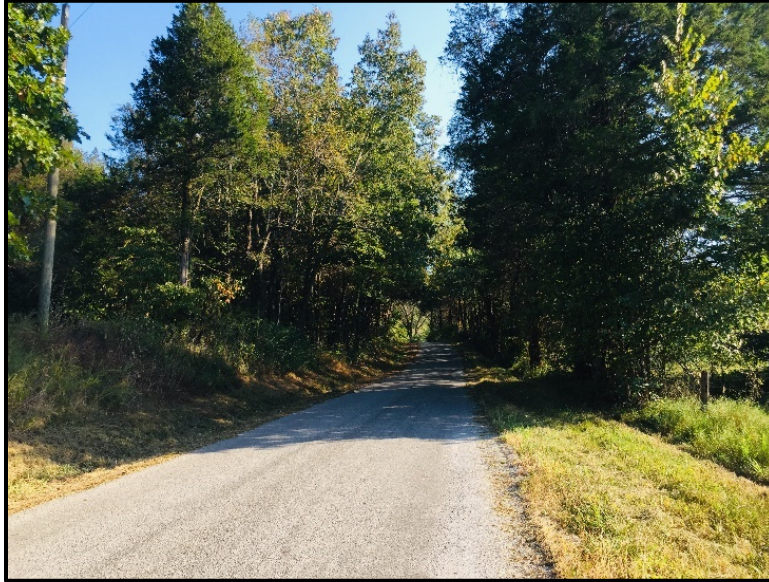
Figure 1.3. Roadside vegetation, which could contribute hazards in the event falling trees block escape routes.
