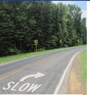
Figure 5. Curve delineation enhancements may include in-lane curve warning pavement markings and chevron signs with retroreflective strips on sign posts. Source: FHWA
