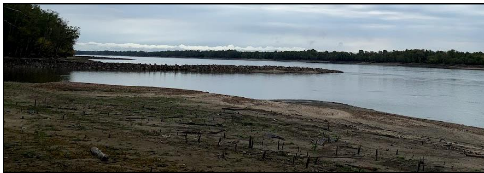
Figure 4.15: The top portion of a wing dam visible in the Mississippi River near Cape Girardeau, MO.
