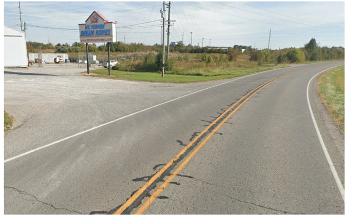
Improper Superelevation Rates Mt. Vernon Dream Home Entrance
