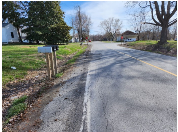
PHOTOS 2 & 3: EXISTING PAVEMENT DAMAGE ON THOMPSONVILLE ROAD
