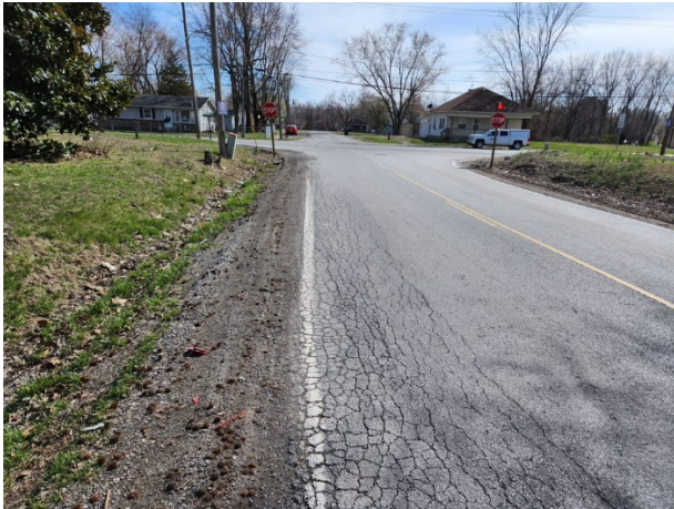
PHOTOS 2 & 3: EXISTING PAVEMENT DAMAGE ON THOMPSONVILLE ROAD
