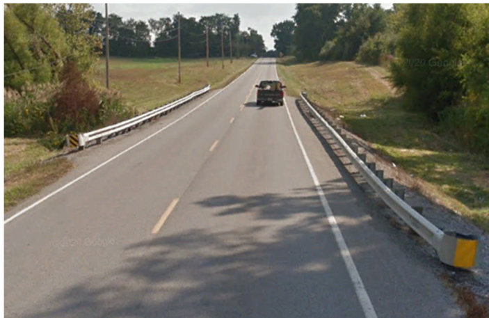
PHOTO 4: EXISTING DEFICIENT GUARDRAIL & TERMINAL SECTIONS
