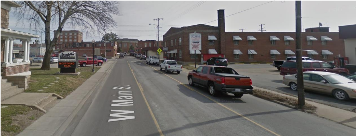
In Benton, the three-lane section of IL 14 between IL 37 and I-57 has an AADT of 12,100 with a truck AADT of 460.
