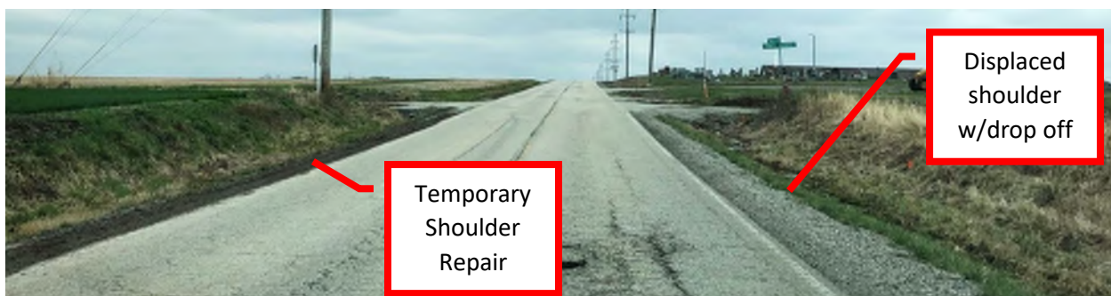
PHOTO 1: SHOULDER REPAIR AT BALDRIDGE RD (MILE 1.0)
