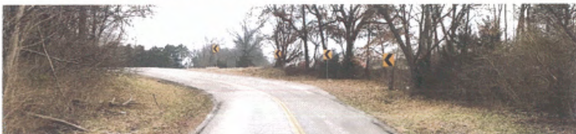
PHOTO 2: NB VERTICAL/HORIZONTAL CURVE (MILE 0.75)
