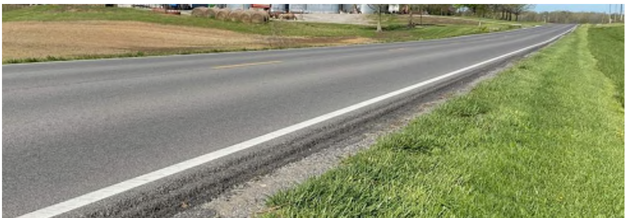
PHOTO 4: SHOULDER DROP OFF WEST OF SEVEN OAKS LN INTERSECTION (MILE 8.40)
