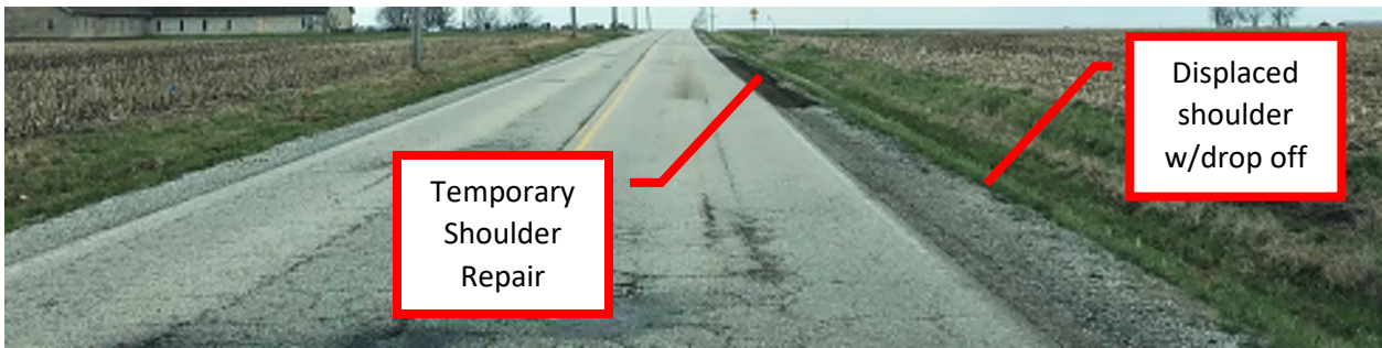
PHOTO 4: DROP OFF AND REPAIR EAST OF RAILROAD CROSSING (MILE 2.55)
