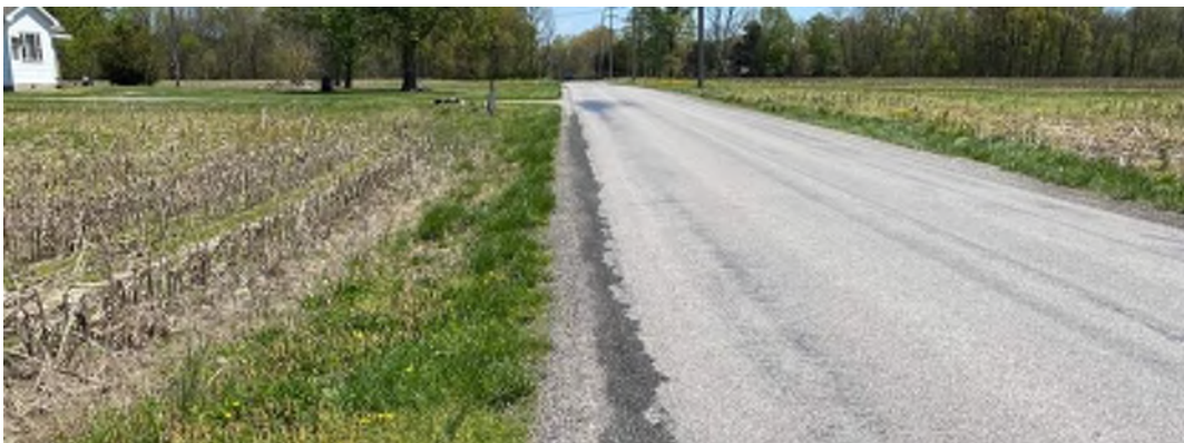
PHOTO 2: SHOULDER REPAIR (MILE 2.45)
