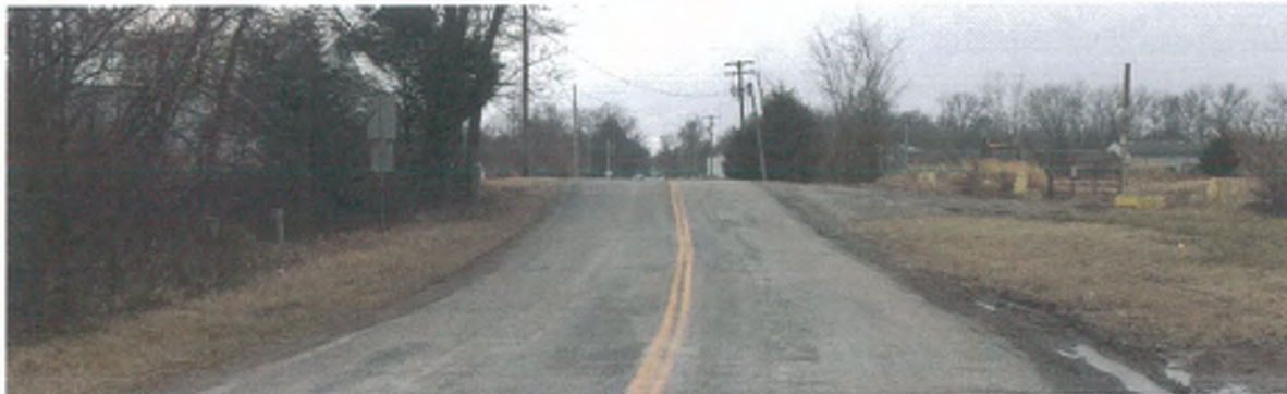
PHOTO 5: SB VERTICAL CURVE (MILE 1.45)
