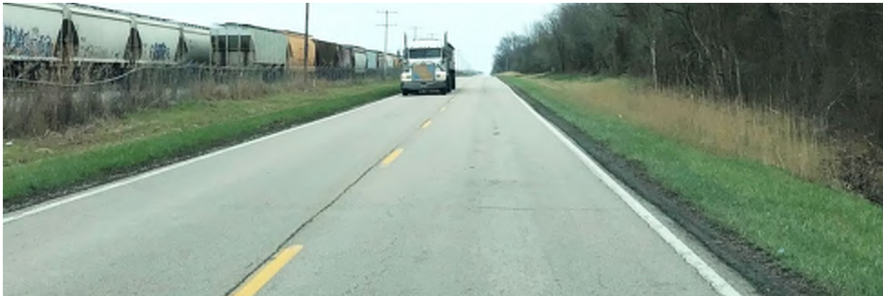
PHOTO 4: MEETING TRUCK EAST OF RAIL TRANSFER TERMINAL (NO AGG SHOULDER)
