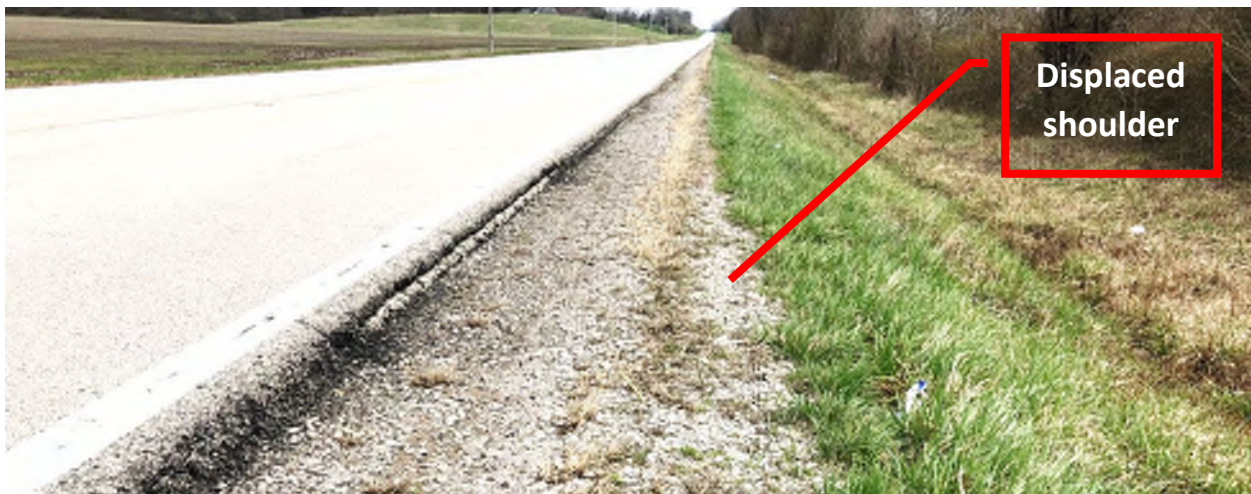
PHOTO 5: DROP OFF EAST OF PYRAMID STATE PARK (TYPICAL CONDITION)
