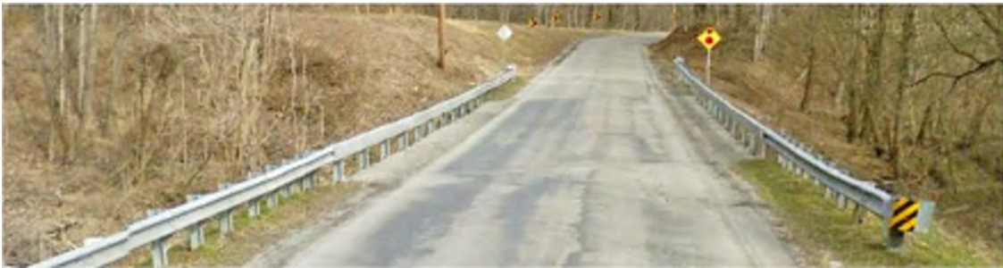
PHOTO 4: EXISTING BRIDGE (MILE 2.85)
