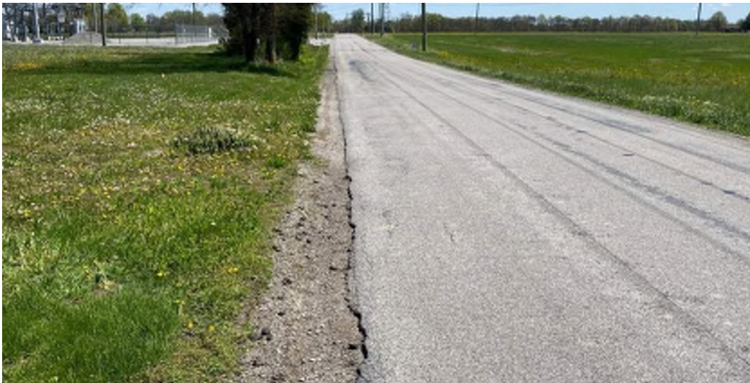
PHOTO 1: EB ROADWAY SECTION (MILE 2.10)
