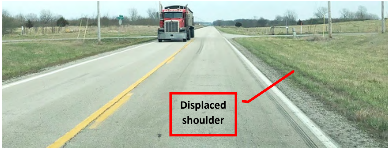
PHOTO 1: EB APPROACH OF TRICO-CUTLER ROAD INTERSECTION (MILE 1.70)
