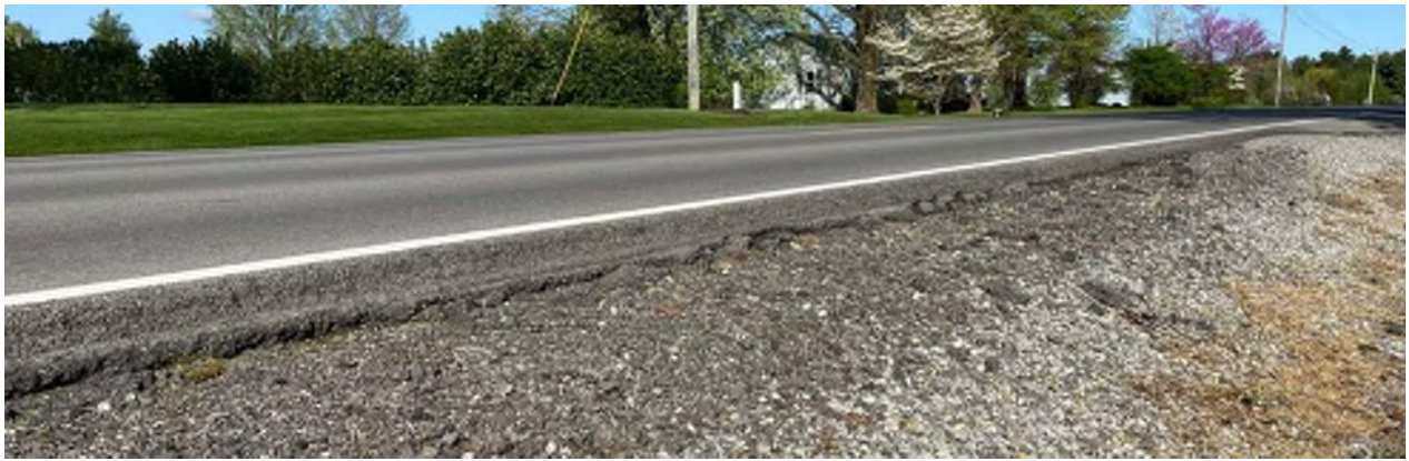
PHOTO 7 SHOULDER DROP-OFF AT SHILOH LANE LN INTERSECTION (MILE 10.38)
