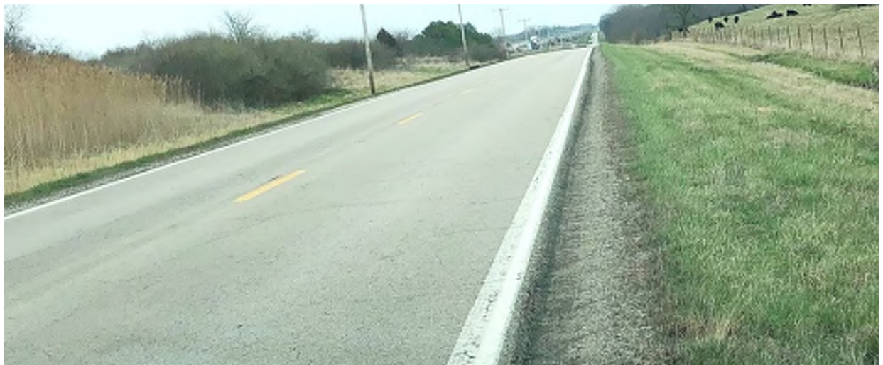
PHOTO 3: DROP OFF WEST OF RAIL TRANSFER TERMINAL
