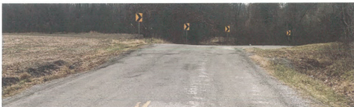
PHOTO 1: SB VERTICAL/HORIZONTAL CURVE (MILE 0.65)
