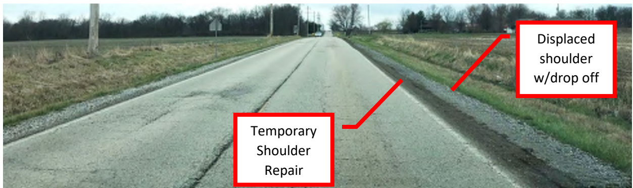
PHOTO 4: DROP OFF AND REPAIR EAST OF RAILROAD CROSSING (MILE 2.55)
