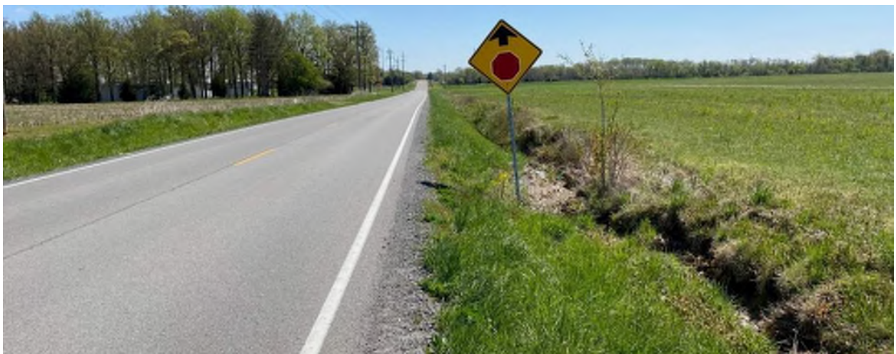
PHOTO 6: ADVANCE WARNING SIGN 1,000 FT FROM THOMPSONVILLE RD (MILE 5.25)
