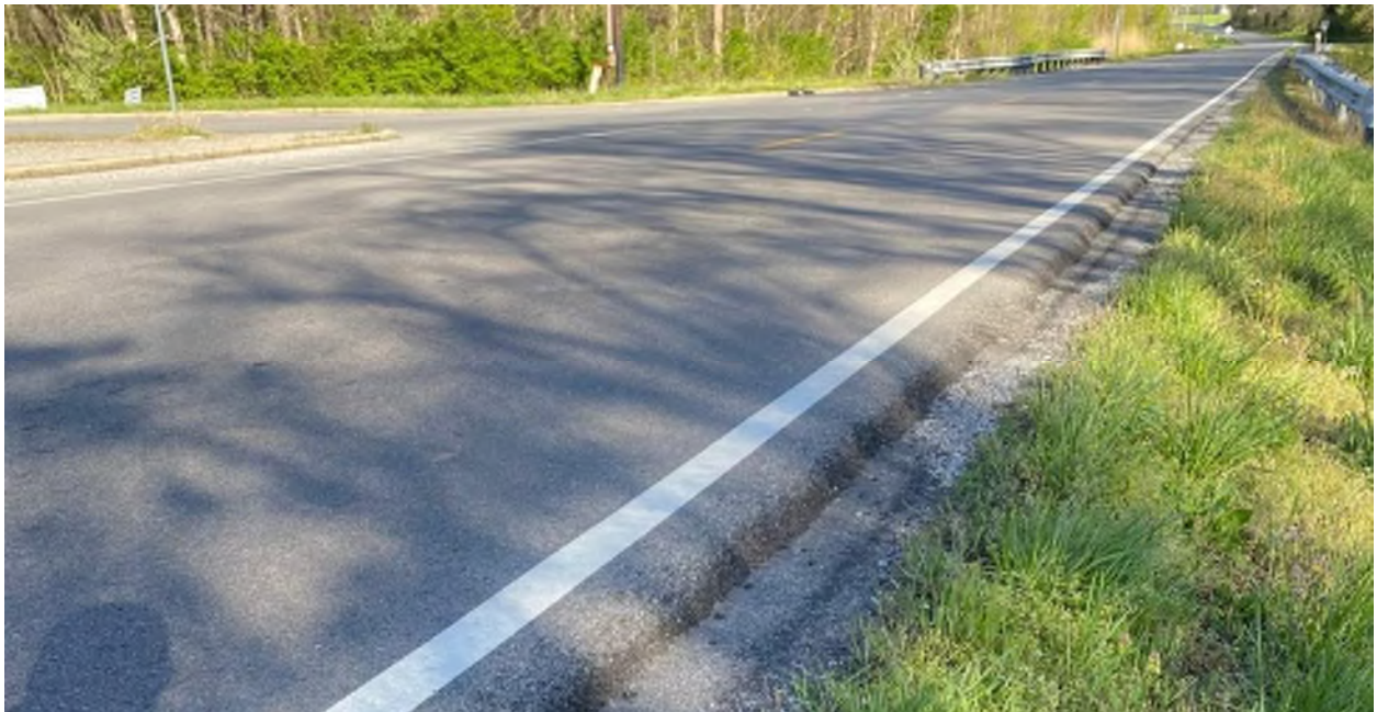
PHOTO 7 SHOULDER DROP-OFF AT SHILOH LANE LN INTERSECTION (MILE 10.38)
