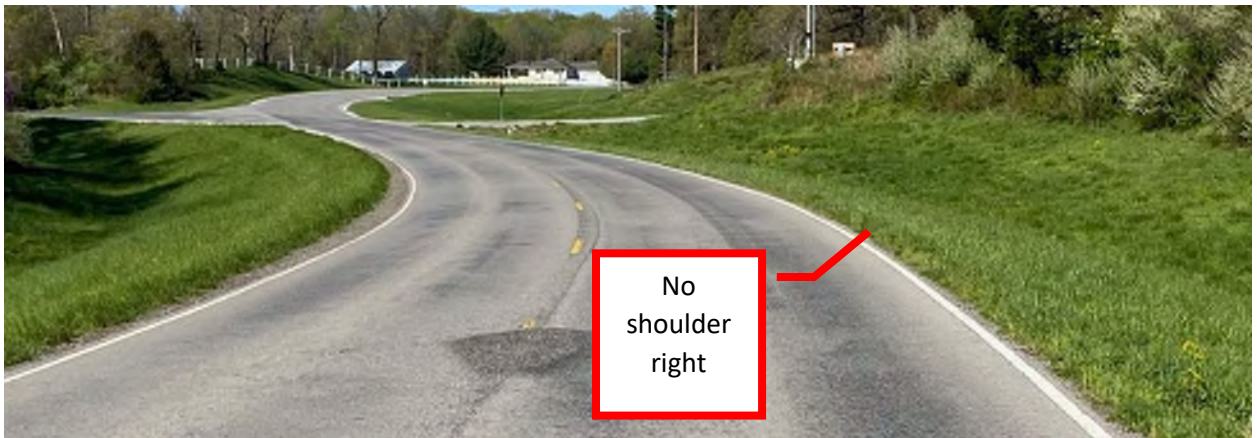
PHOTO 4: SHOULDER DROP OFF WEST OF SEVEN OAKS LN INTERSECTION (MILE 8.40)
