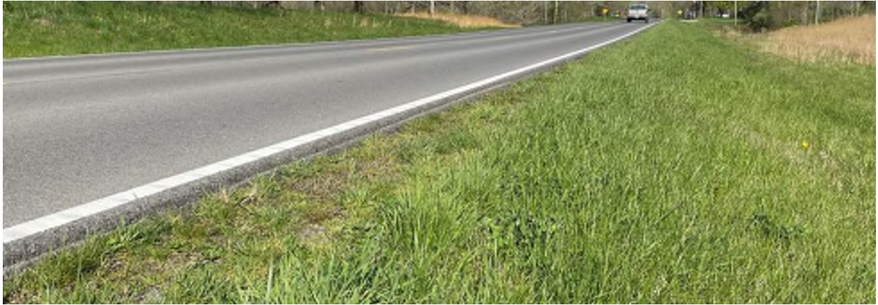
PHOTO 6: SHOULDER DROP-OFF EAST OF E. BOYD RD INTERSECTION (MILE 9.95)
