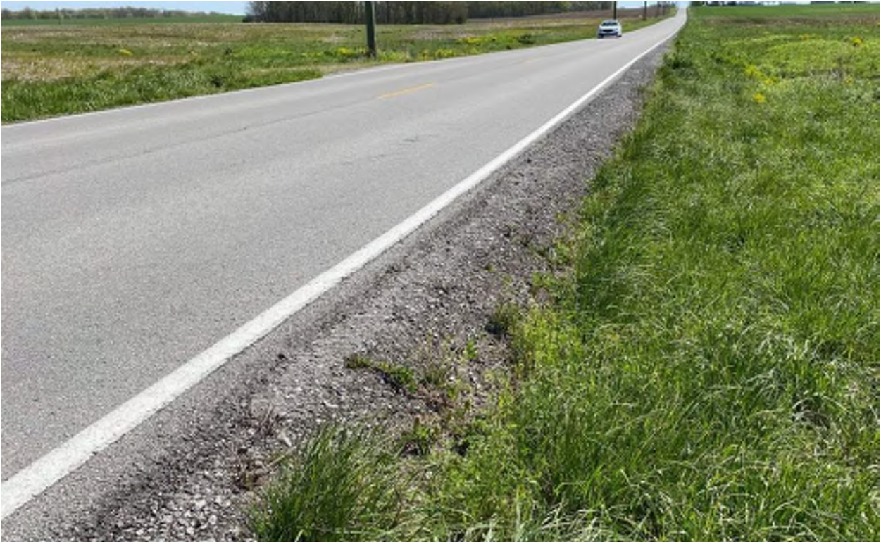
PHOTO 4: SHOULDER DROP OFF/ REPAIR (MILE 3.72)
