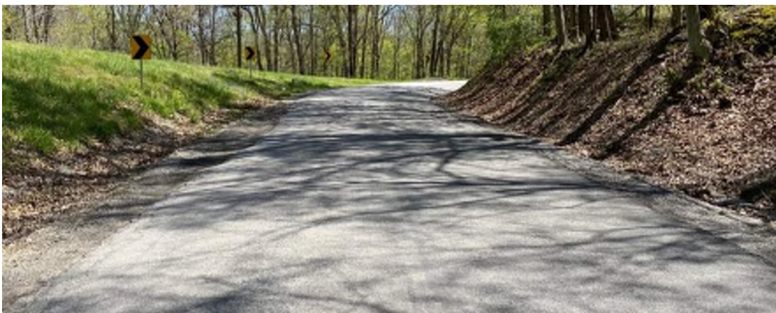
PHOTO 5: HORIZONTAL CURVE (MILE 2.95)
