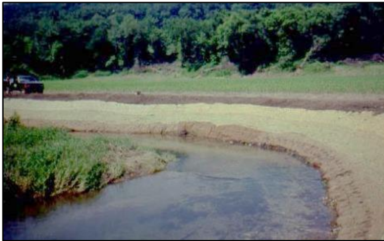
Figure 4.16 - A regraded streambank that has been seeded
