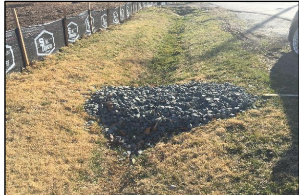
Figure 4.8 Stone Check Dam
