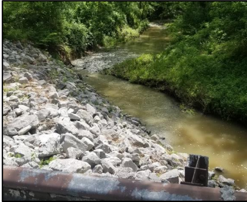
Figure 4.14 - Rip Rap along Indian Creek
