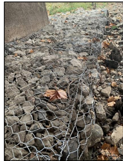
Figure 4.15 – Gabion Baskets along Crab Orchard Creek
