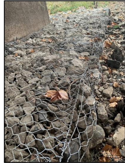
Figure 5.14 – Gabion Baskets along Western Crab Orchard Creek
