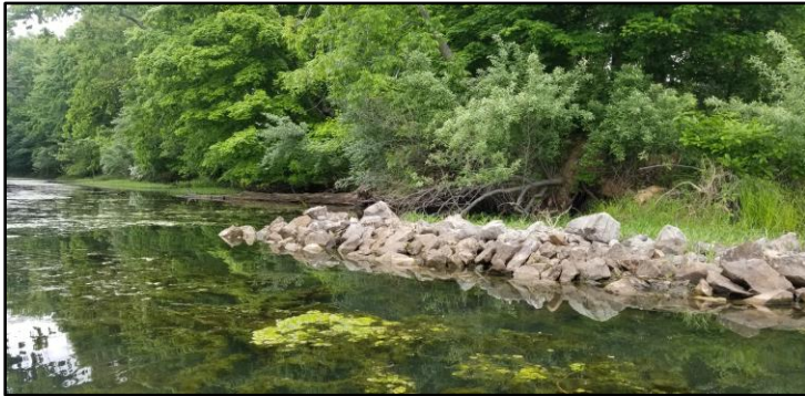
Figure 5.13 - breakwater structures at Lake Kinkaid
