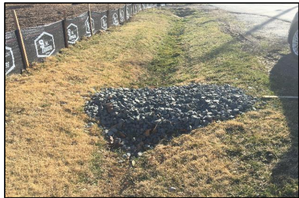
Figure 5.11 Stone Check Dam
