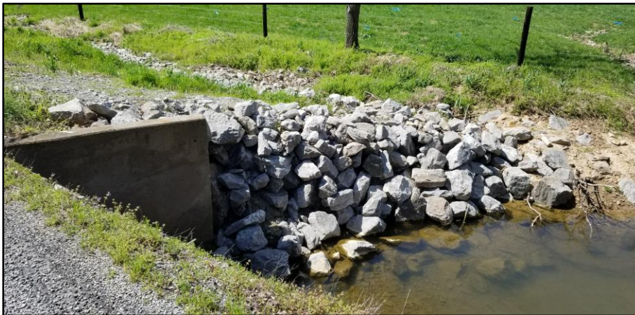
Figure 5.12 - Rip Rap along a stream in the Kinkaid Creek Watershed
