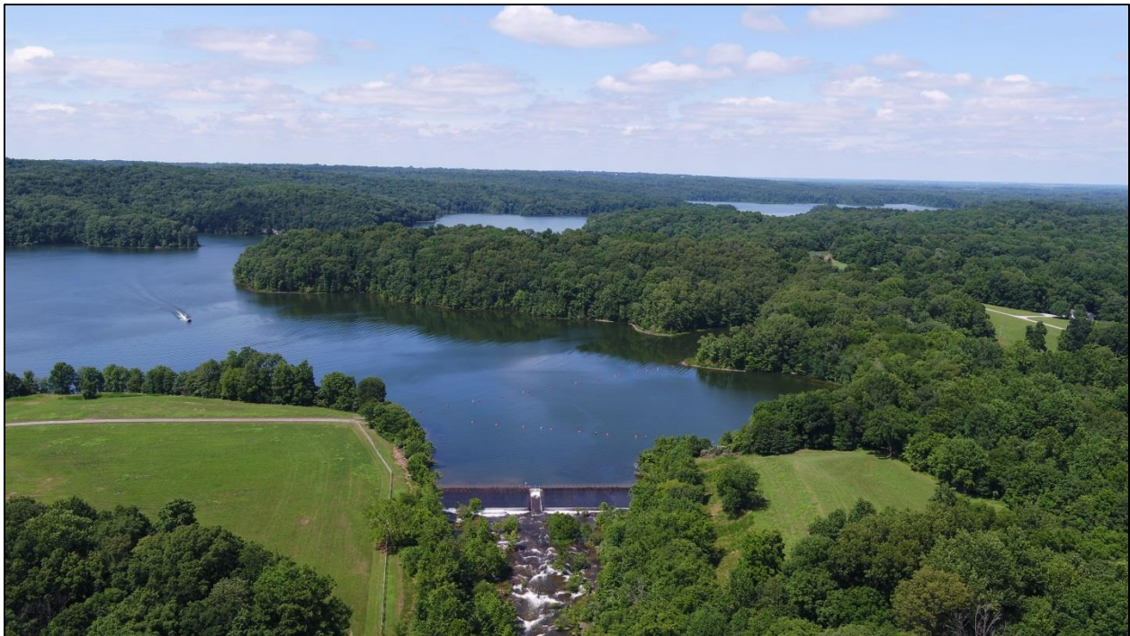
Figure 2.2- Kinkaid Lake Spillway- North Facing
