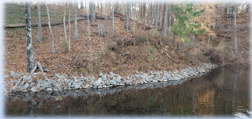
Bank stabilization at Spring Arbor Lake
