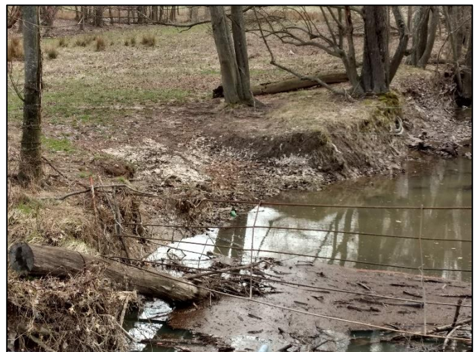
Figure 44- Location in Need of Livestock Crossing Structure
